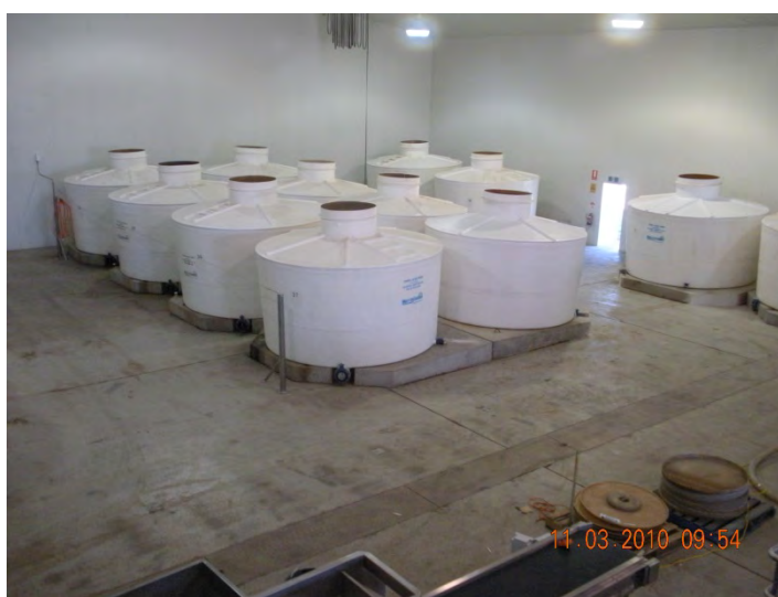
Figure 1: New FRP tanks on sloping plinths being fitted out. Note power line on left-hand-side of tank.
