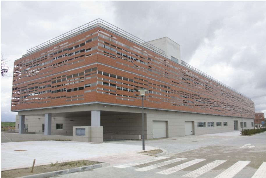
CITOLIVA and CEAS instalations in GEOLIT
